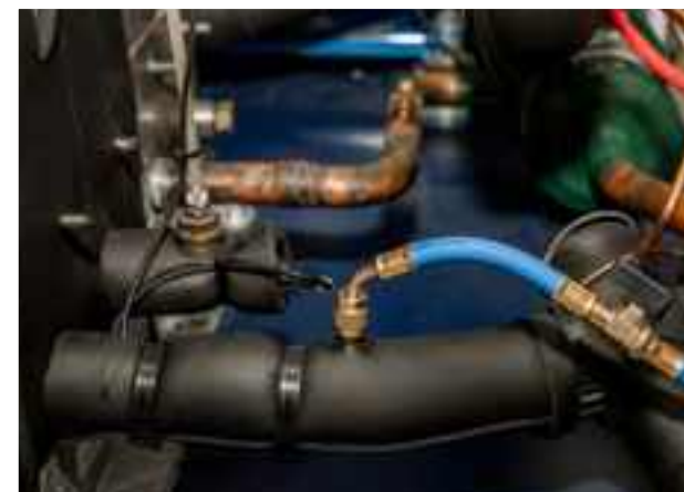
Connection hoses with ball valves for quick closing and opening of refrigerant flow.
